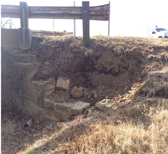
PHOTO 1 Description Erosion to the North slope at the West bridge end.
