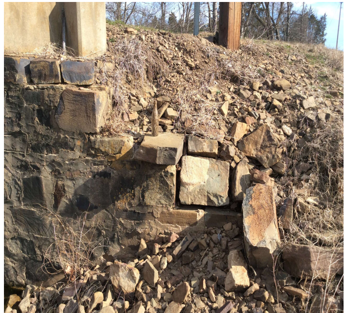
PHOTO 2 Description Southeast wing has Displaced stones.
