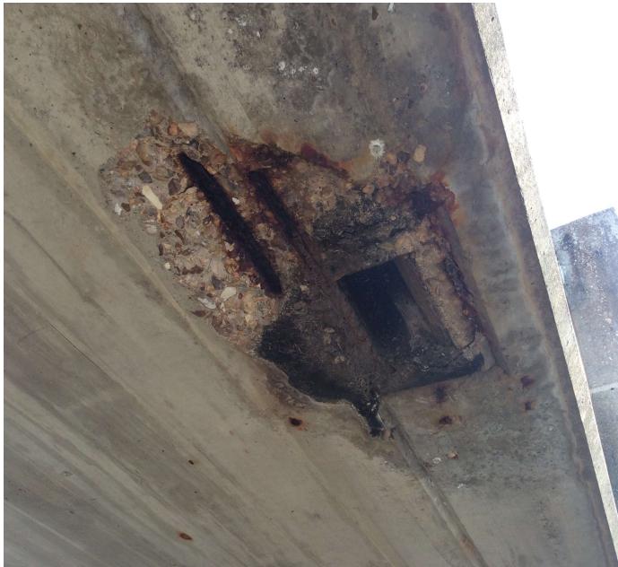
PHOTO 1 Description Spalling with exposed reinforcing steel adjacent to deck drain on Right side of span #3.
