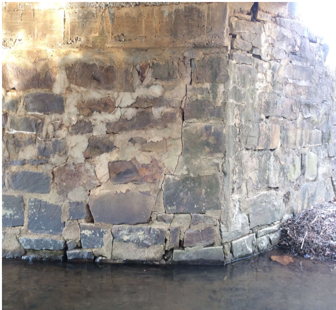
PHOTO 1 Description Vertical crack in the Right side of the West abutment breast wall.
