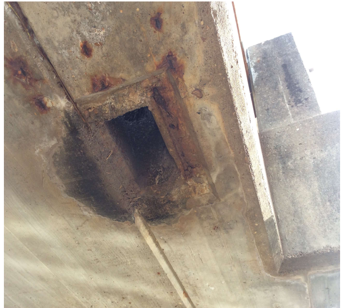
PHOTO 2 Description Spalling with exposed reinforcing steel adjacent to deck drain.
